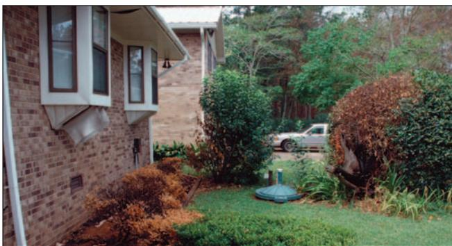
FIGURE 5. A row of foundation shrubs ignited in front of this house during a wildfire. Notice how the vinyl siding around the windows and the vinyl soffit vents were damaged, but the brick was not.
