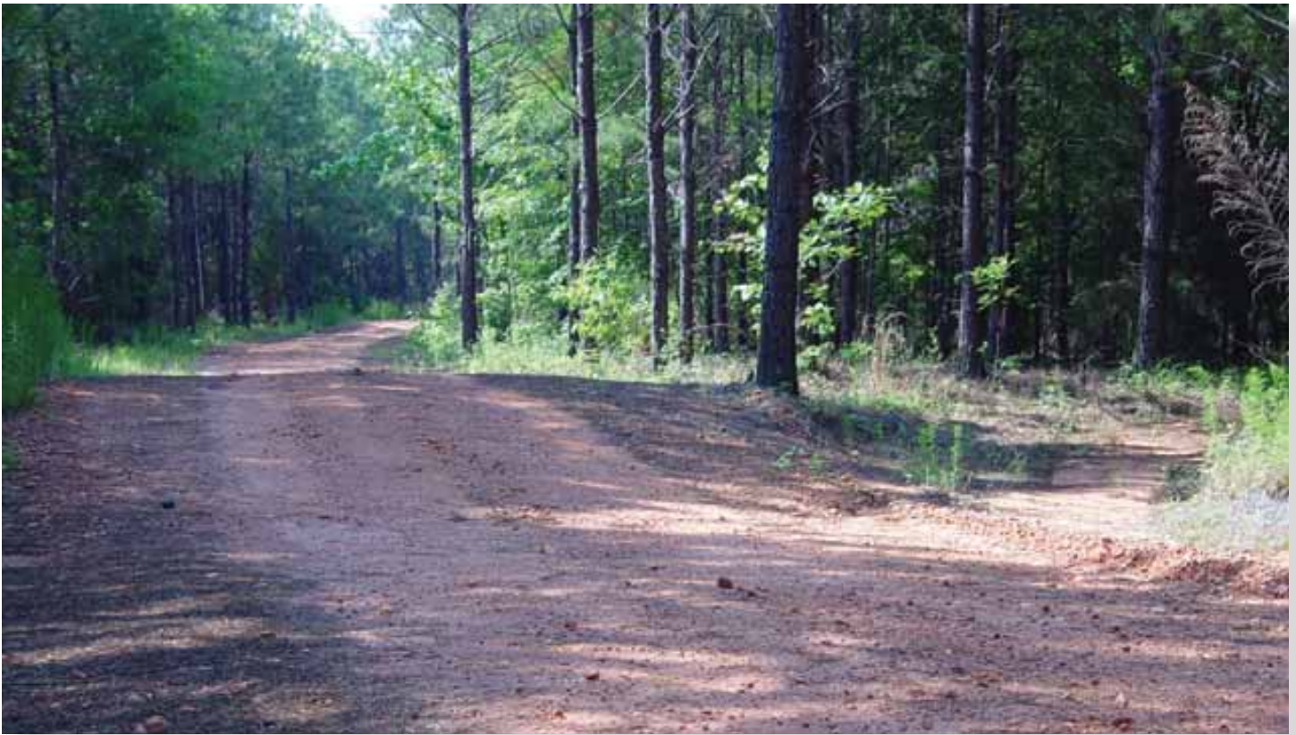
A broad-based dip used to divert water from the road surface.
