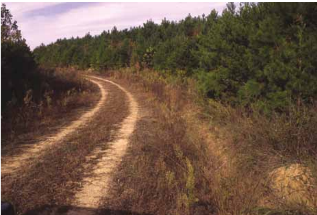
A well-designed road with a gentle grade; crowned, rock surface; drainage; daylighting; and vegetation for stabilization.
