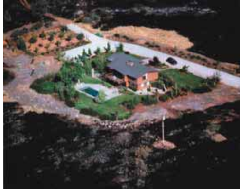
The pre-fire activities implemented by this homeowner included a green and well maintained landscape, reduction of wild vegetation around the perimeter of the property, a fire-resistant roof, and a good access road with a turnaround area. As seen in the photo, these pre-fire activities were effective.
