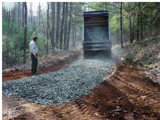
*Geotextile filter fabric installed on the left, and gravel being applied atop of the geotextile on the right.*
