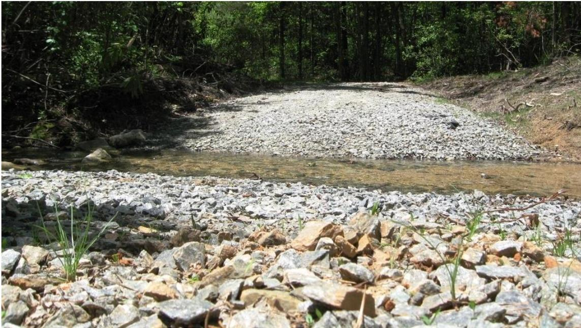
*This ford crossing was installed to replace an improper crossing of logs, boulders, and soil. The stream is now open and free to flow, without excessive fill material blocking the channel.*
