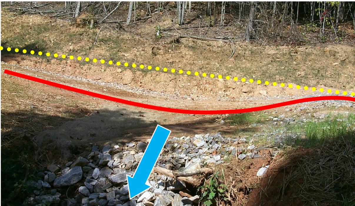
*This is a side view of a broad-based dip. The dotted line shows the original road grade.
