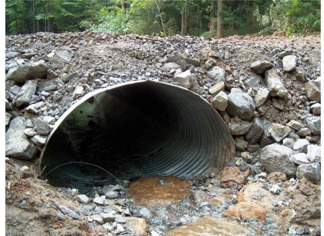
*This is an oval, steel culvert that was installed in this stream for a road crossing. The flat bottom provides better water flow and allows improved fish passage.*
