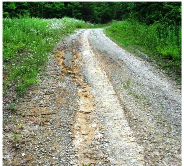
*This road needs re-grading, installation of water control diversions, and significant groundcover establishment work.*
