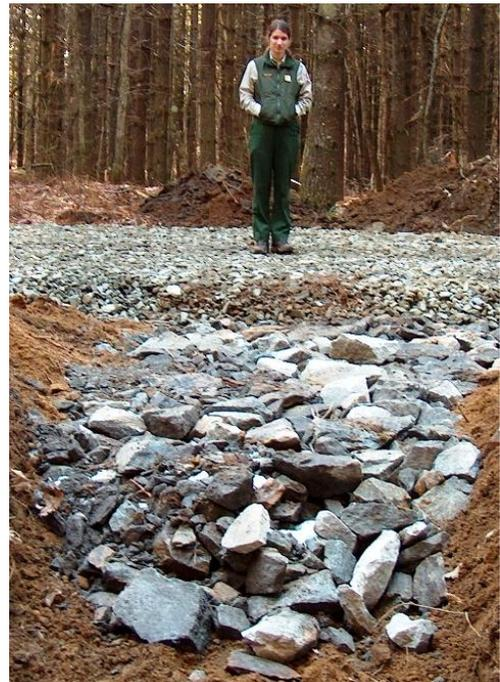
*Large stones are placed into a catch basin for draining stormwater runoff off the gravel road.*
