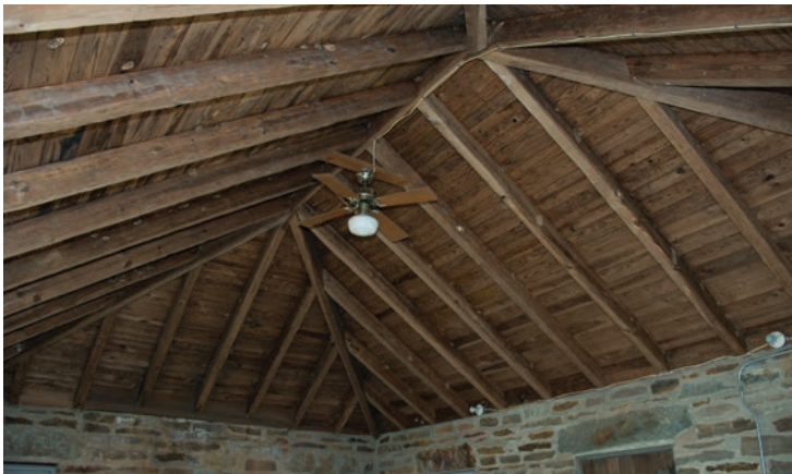
Vaulted ceiling at the Flagg Mountain tower
