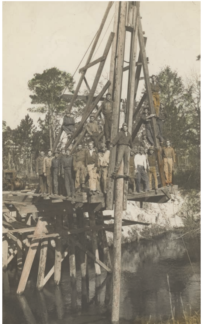
CCC company driving bridge piling, Mobile County
