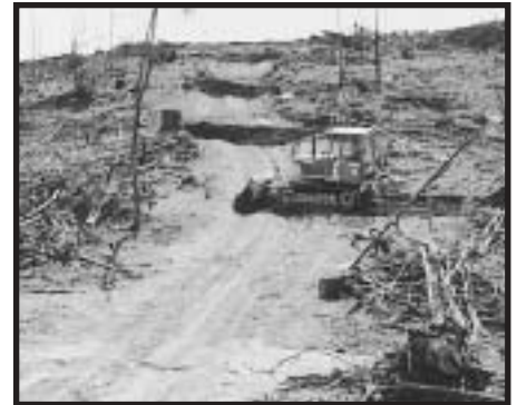
Installing water bars and/or turnouts prevent road erosion on harvested site.
