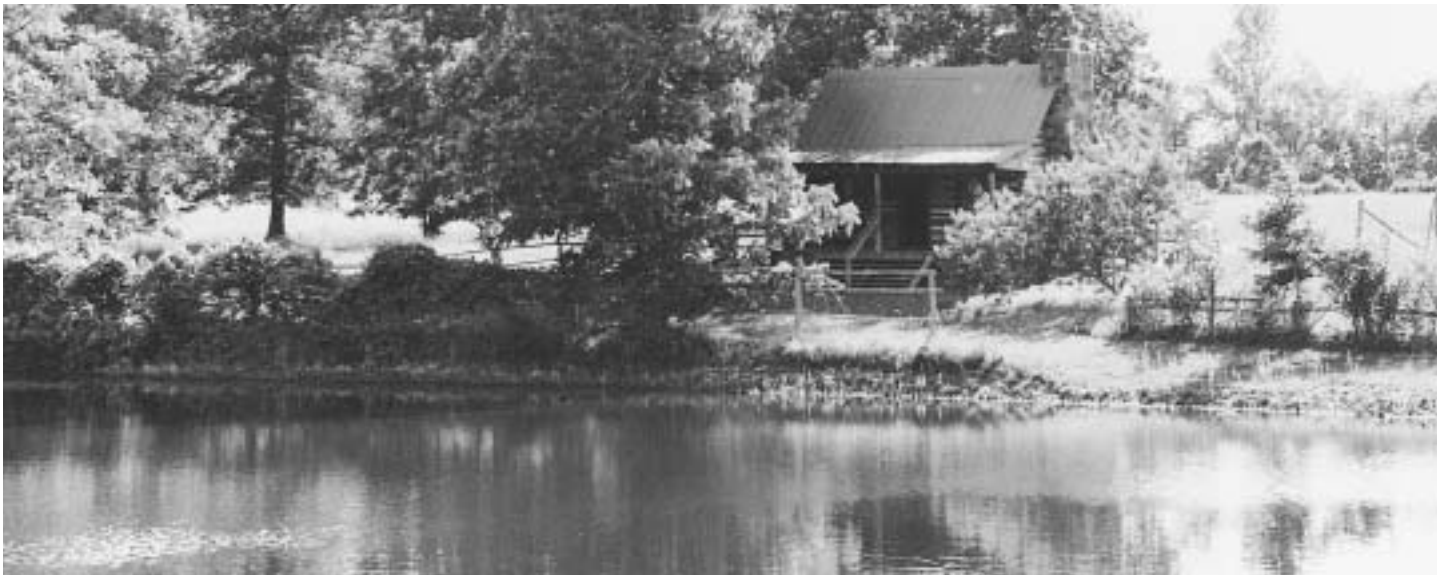
Dr. Mims cut the logs and laid the rocks to build this cabin.
