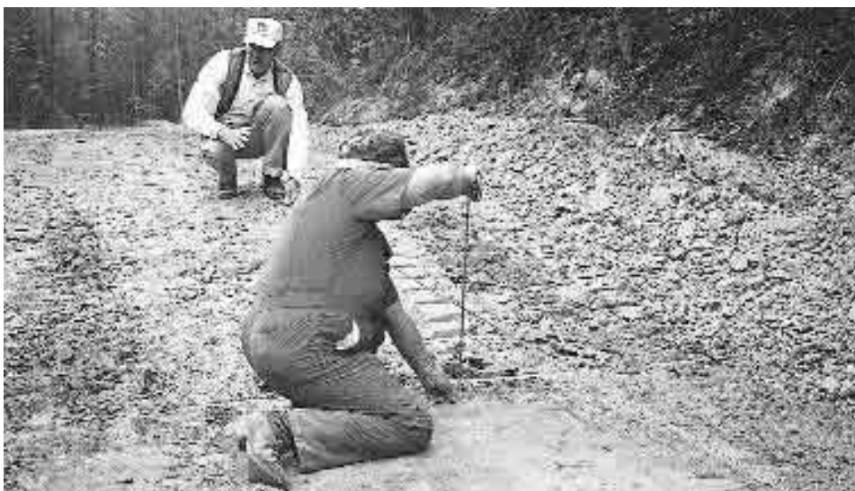
Dr. Richard Brinker (rear of photo), dean of the School of Forestry and Wildlife Sciences, assists the road crew in laying out a broad-based dip for demonstration purposes.
