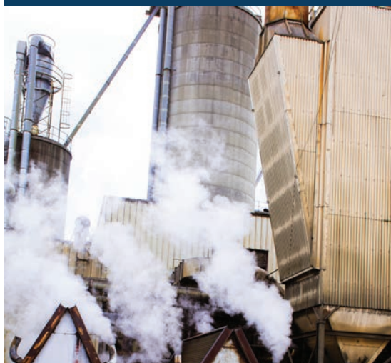
Energy generated provides the heat needed for paint dryers and the dry kilns.
