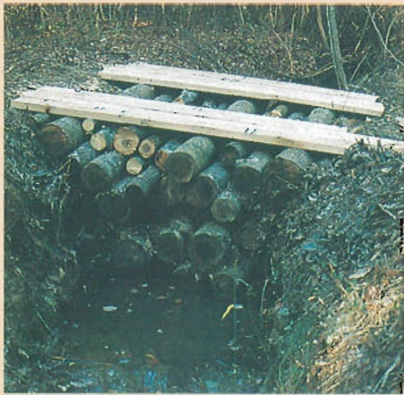
A log crossing is temporary and must be removed when activity (such as a logging operation) is completed.
